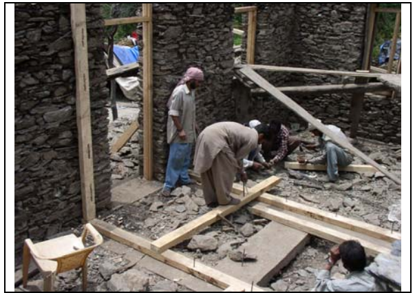
Dhajji wall anchored to Band & UCR Wall
