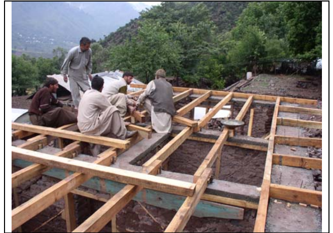
Anchoring roof deck to Eave Band
