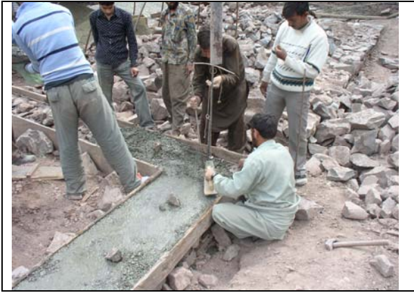
Shear keys on top of RC Band
