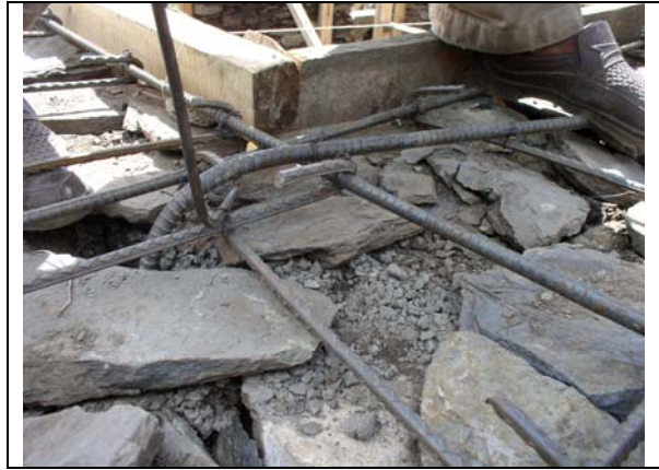
Connecting vertical reinforcement to RC Band
