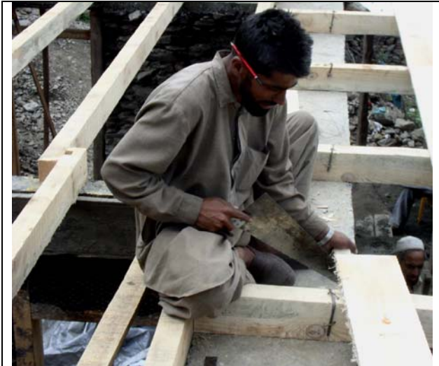
Installation of attic floor framing
