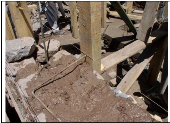
Dhajji wall anchor to UCR wall
