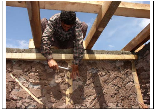
Chicken Wire Mesh confinement on Dhajji wall
