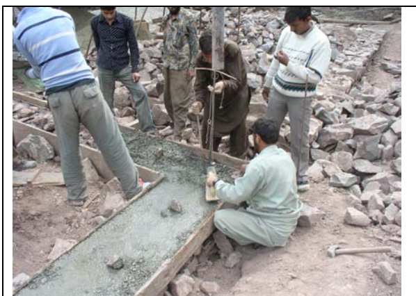
Shear keys on top of RC Band
