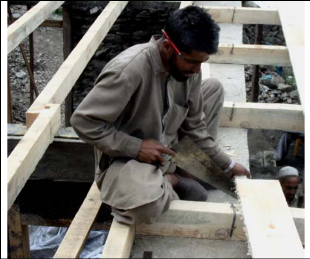
Installation of attic floor framing
