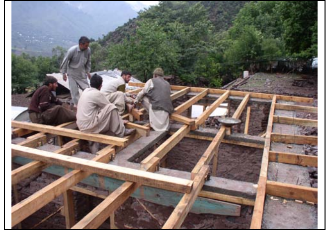
Anchoring roof deck to Eave Band
