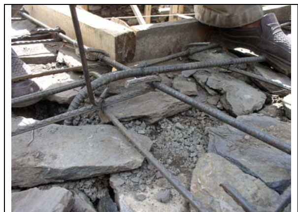
Connecting vertical reinforcement to RC Band
