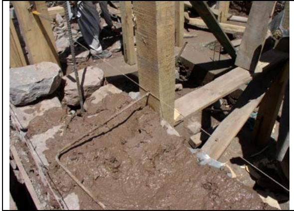
Dhajji wall anchor to UCR wall
