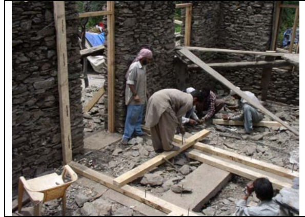
Dhajji wall anchored to Band & UCR Wall
