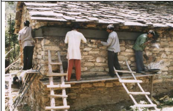
Finishing the Seismic Belt of Ferrocement
