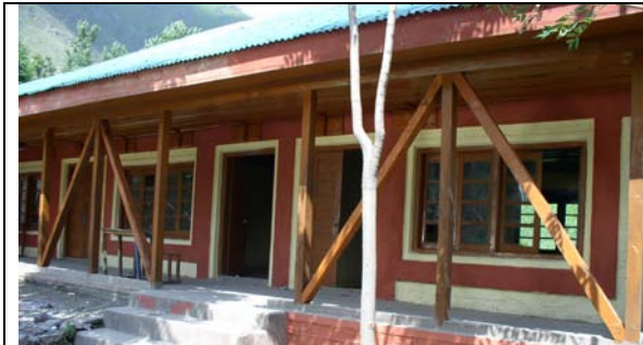
Retrofitting vernacular school building in Kashmir
