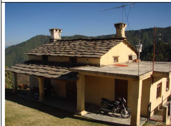
RC extension to a small, old, Vernacular house
