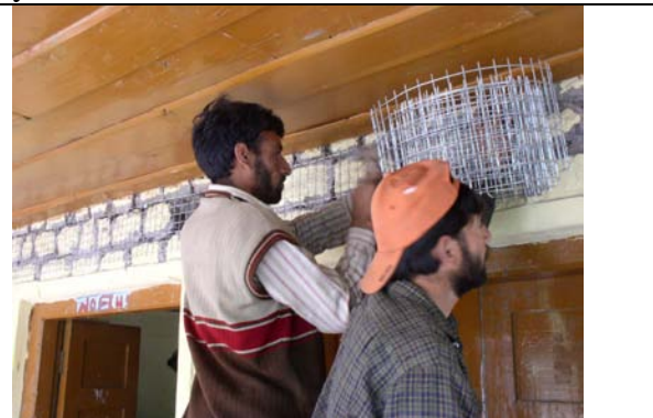
Installing reinforcing weld mesh for the Seismic Belt
